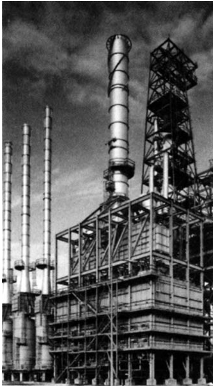
Platformer fired heaters are prominent features of the Marathon Oil Company 200,000 BPD Garyville Refinery in Louisiana.
