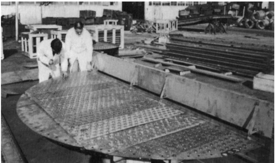
A typical stainless steel valve cap tray that might be used in a fluid catalytic cracker gas treating plant.
